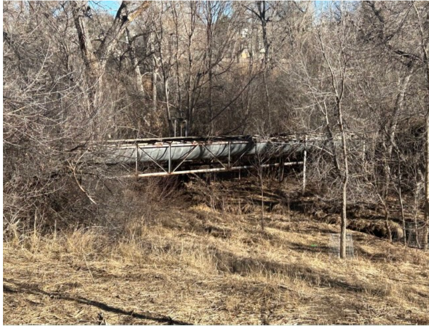
City Ditch Flume over Lee Gulch in Ridgewood Park in Littleton. After 2026, this flume will never carry Ditch water again.
