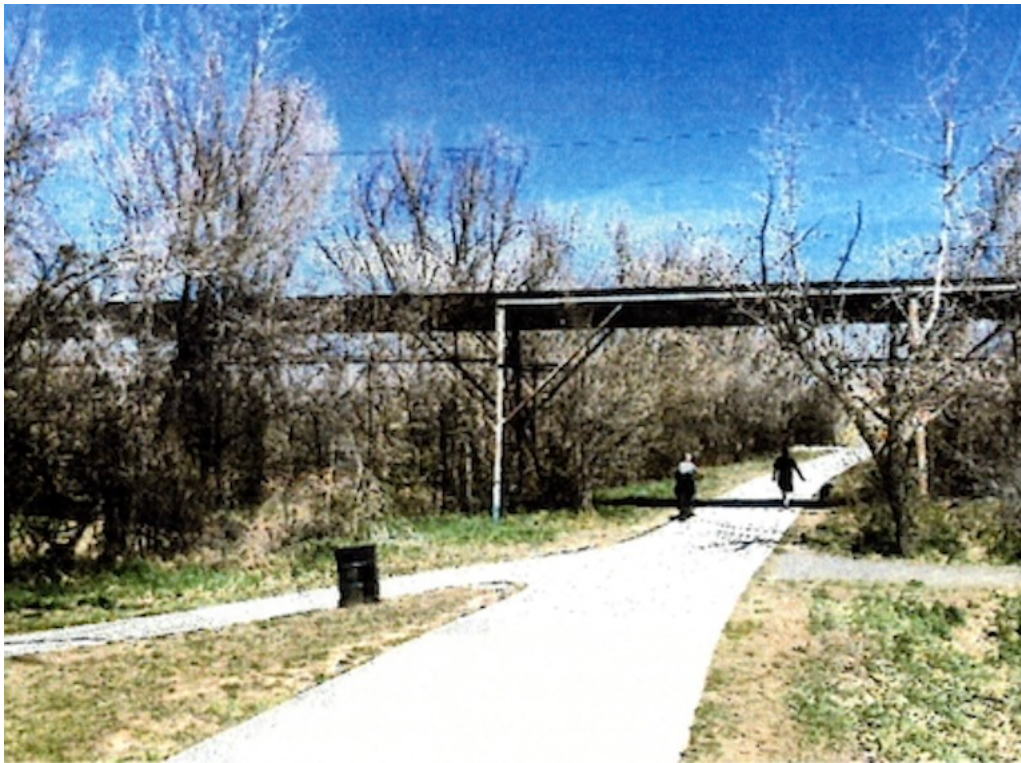
City Ditch Flume over Big Dry Creek in Belleview Park in Englewood. This Flume will continue to carry Ditch water but the Flume is covered and flowing water is not visible.
